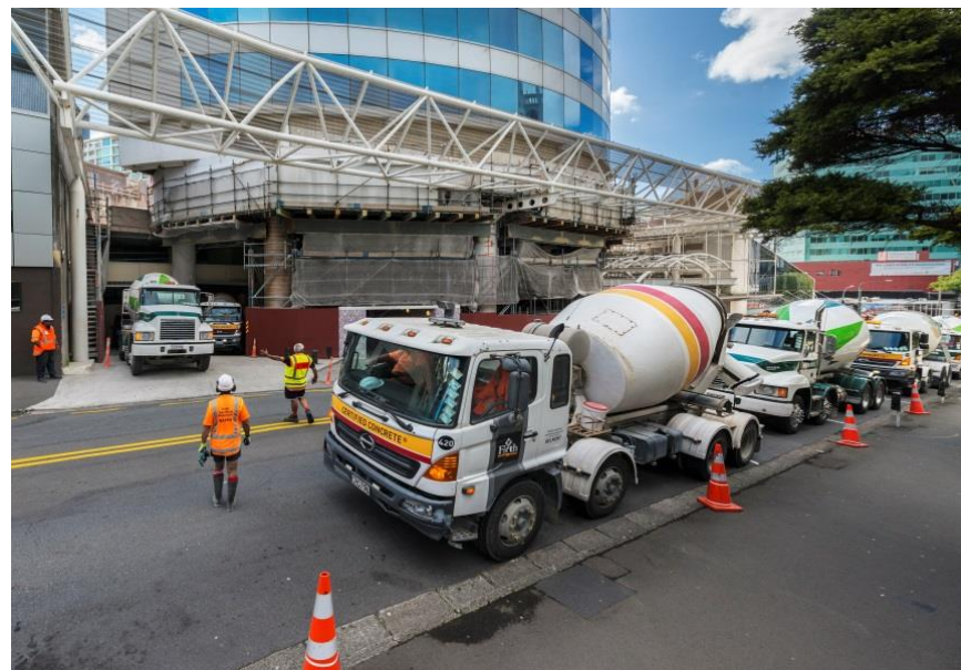
Major foundation concrete pour: 79 trucks, 366 cubic metres
